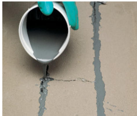
Repairing a crack in cement screed with Eporip
