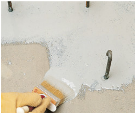
Applying Eporip by brush on construction joint
