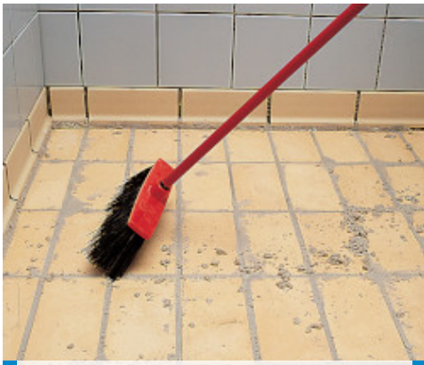
Removing the excess Kerapoxy SP with a broom
