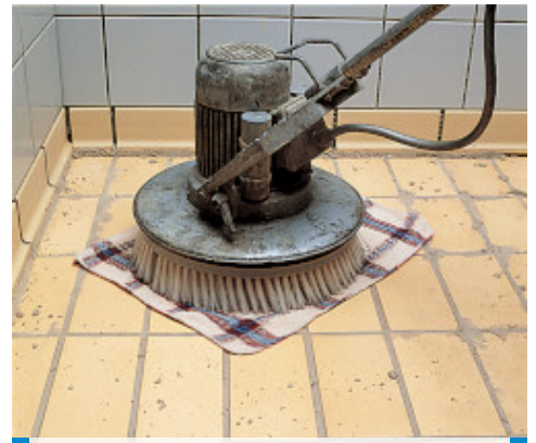
Cleaning with alcohol and a cloth using a rotary-disk type power float
