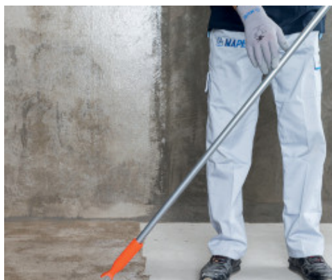
Application of Primer SN on the substrate
