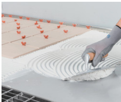
Applying the floor or wall covering with Kerapoxy Easy Design
