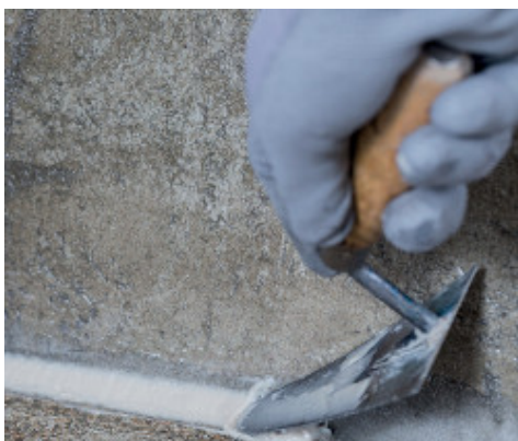
Forming fillet joints
