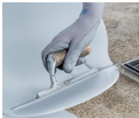
Application of Mapegum EPX
