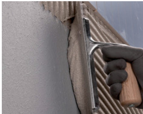
Installing floor covering using Ultramastic III
