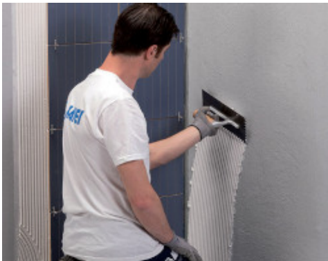
Installing wall covering using Keraflex Maxi S1
