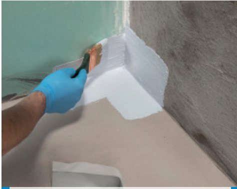
Application of a 90° Mapeband PE 120 corner piece using Mapegum WPS
