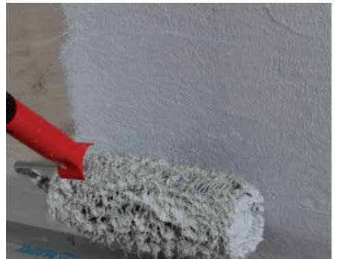
Application of Mapegum WPS with a roller
