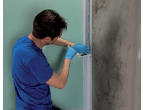
Application of Mapeband PE 120 using Mapegum WPS
