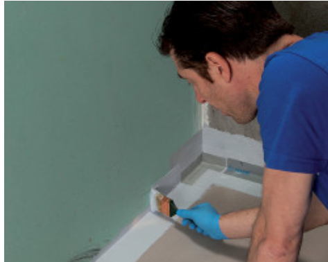
Application of Mapeband PE 120 using Mapegum WPS
