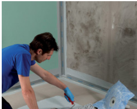
Application of a Drain Vertical fitting using Mapegum WPS
