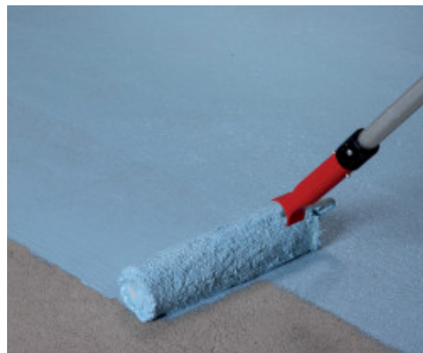
Application of the first coat of Mapelastic AquaDefense on a screed
