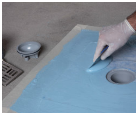
Impregnating Drain Vertical fabric with Mapelastic AquaDefense
