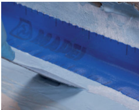
Application of Mapeband on a wall-floor fillet joint with Mapelastic AquaDefense
