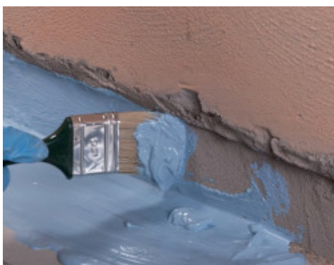
Application of Mapelastic AquaDefense by brush between floor and wall before applying Mapeband
