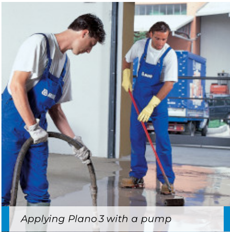
Using a roller on freshly applied Plano3
